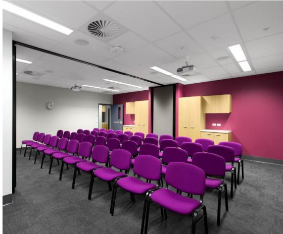
Figure 22: Acoustic tile ceiling suitable for Offices and Conference rooms
