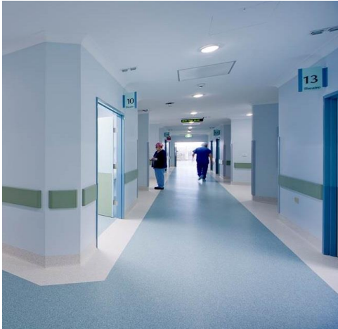
Figure 27: Seamless flooring and covered skirting in clinical areas such as Operating Unit are integral and covered
